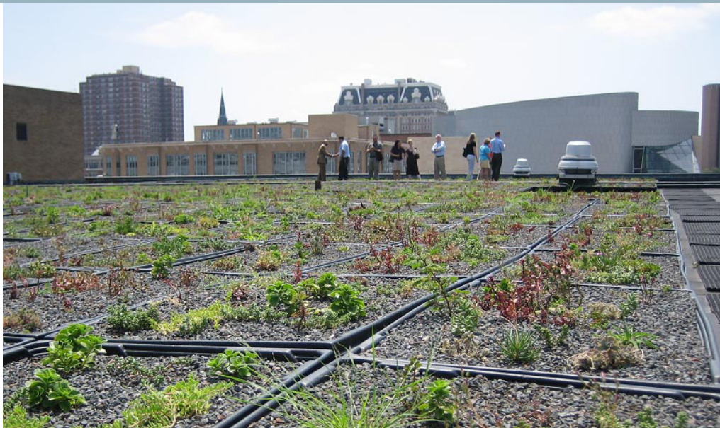
Angelos Law Center Green Roof
