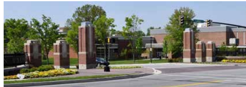
The new Osler Drive bridge and Towsontown Gateway define the campus edges
