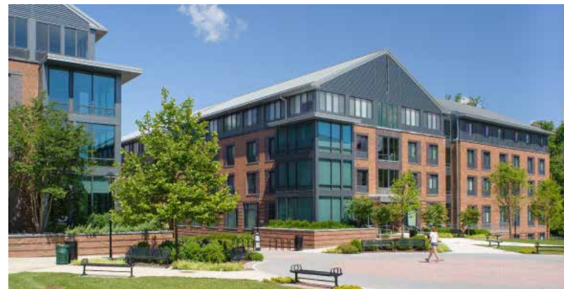
Phase 2 housing in the West Village added over 600 beds
