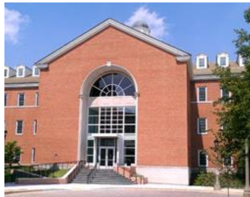
Front entrance of Administration Building
