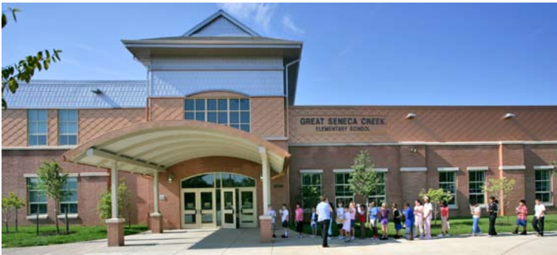
Great Seneca Creek Elementary School, Montgomery County - LEED Silver
